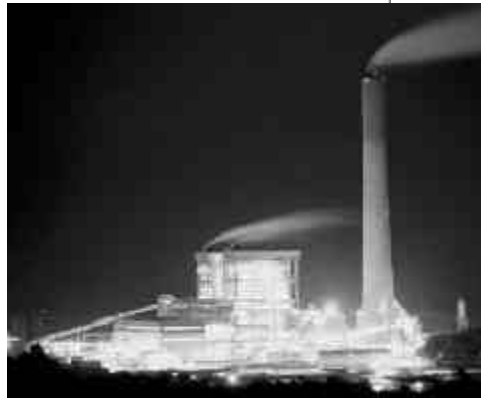
The 1200-MW Sual coal-fired power plant in Pangasinan.
